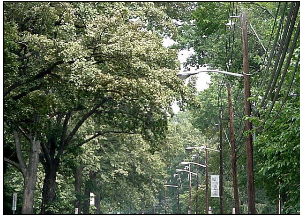
Properly located & maintained, trees and wires can co-exist.
